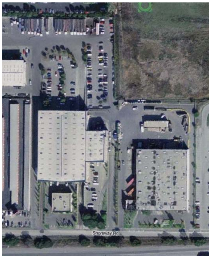
Figure 2-2. SRDC Facility Overview
